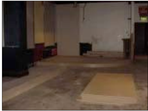
The rear raised floor area being constructed
