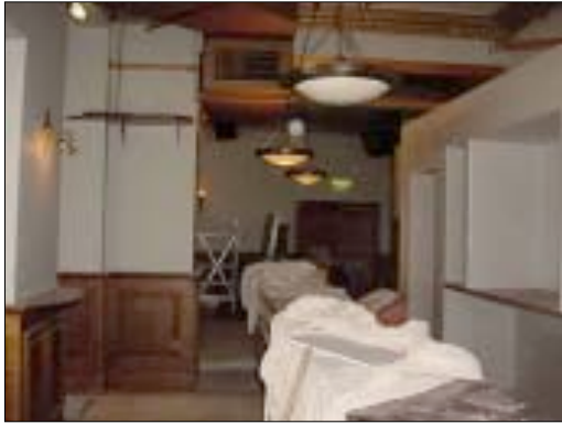
The new bar taking shape
