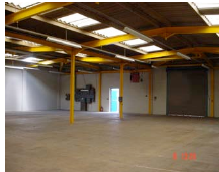
Facing Emergency Exit door. Electric Power by Emergency Exit.
