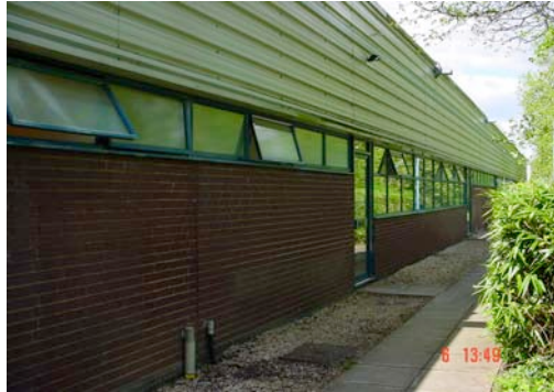
Altered Office windows with brickwork below
