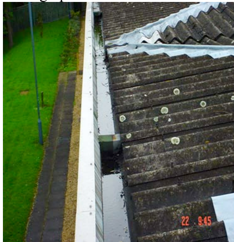
Gutter to Front elevation
