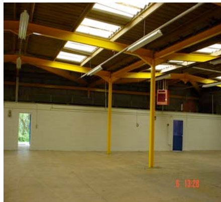
Open Area facing Offices [ view through to Foyer]
