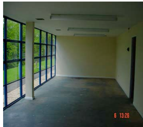
Office with metal windows & glazing to floor level.
