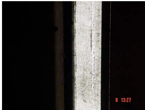
GRP roof light – note bright line running in trough of light.
