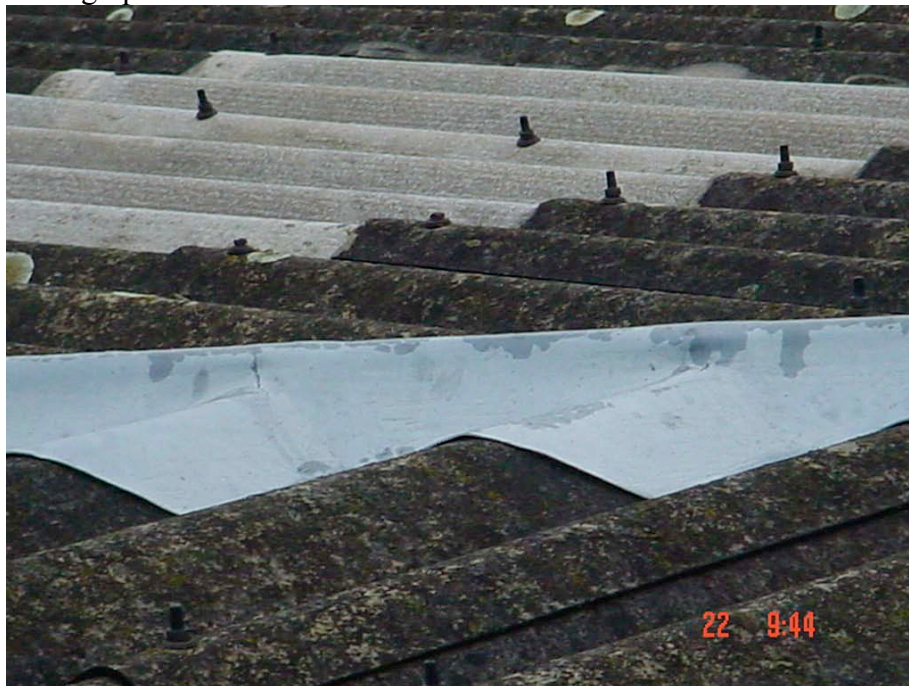
Hip to Row 2. [over Foyer/Toilets] Lead hip with split on ridge. [ approximately \frac{1}{4} up from left hand side]
